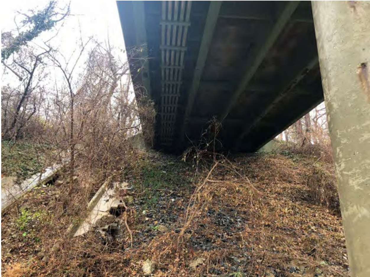
Figure 14 – Utility Conduits Supported by the Existing Superstructure
