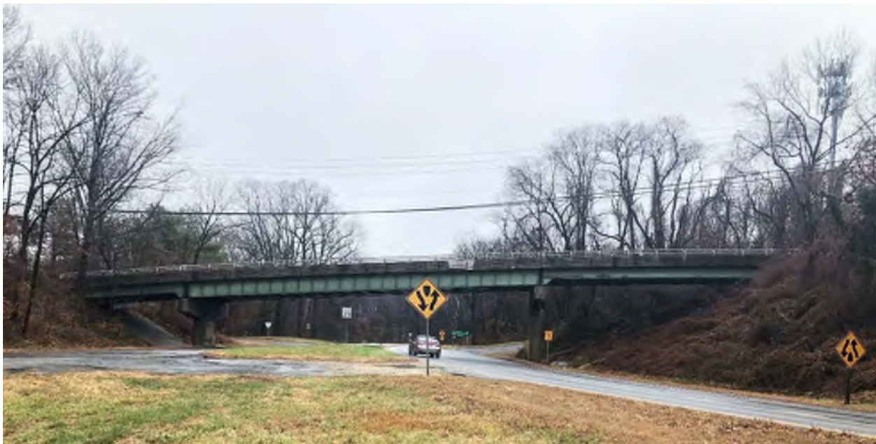
Figure 15 – Overhead Utility Line on West Side of the Existing Structure
