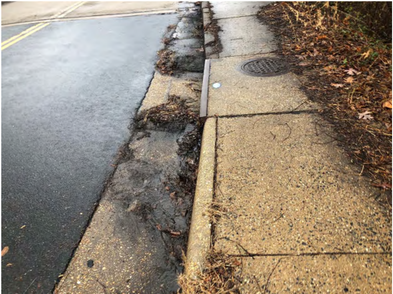
Figure 13 – Drainage Inlets on South End of the Bridge
