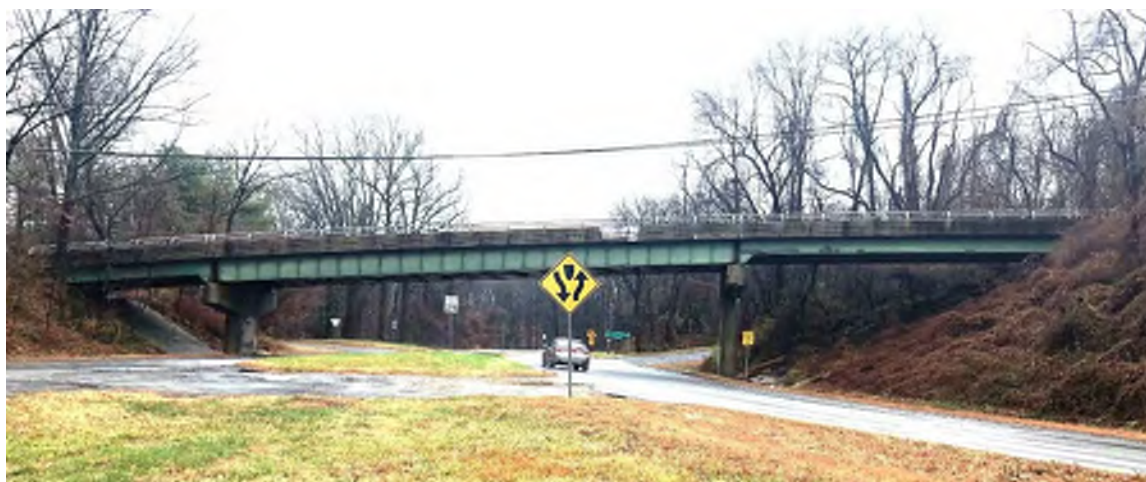
Figure 2 – Elevation View of Existing Structure Looking East
