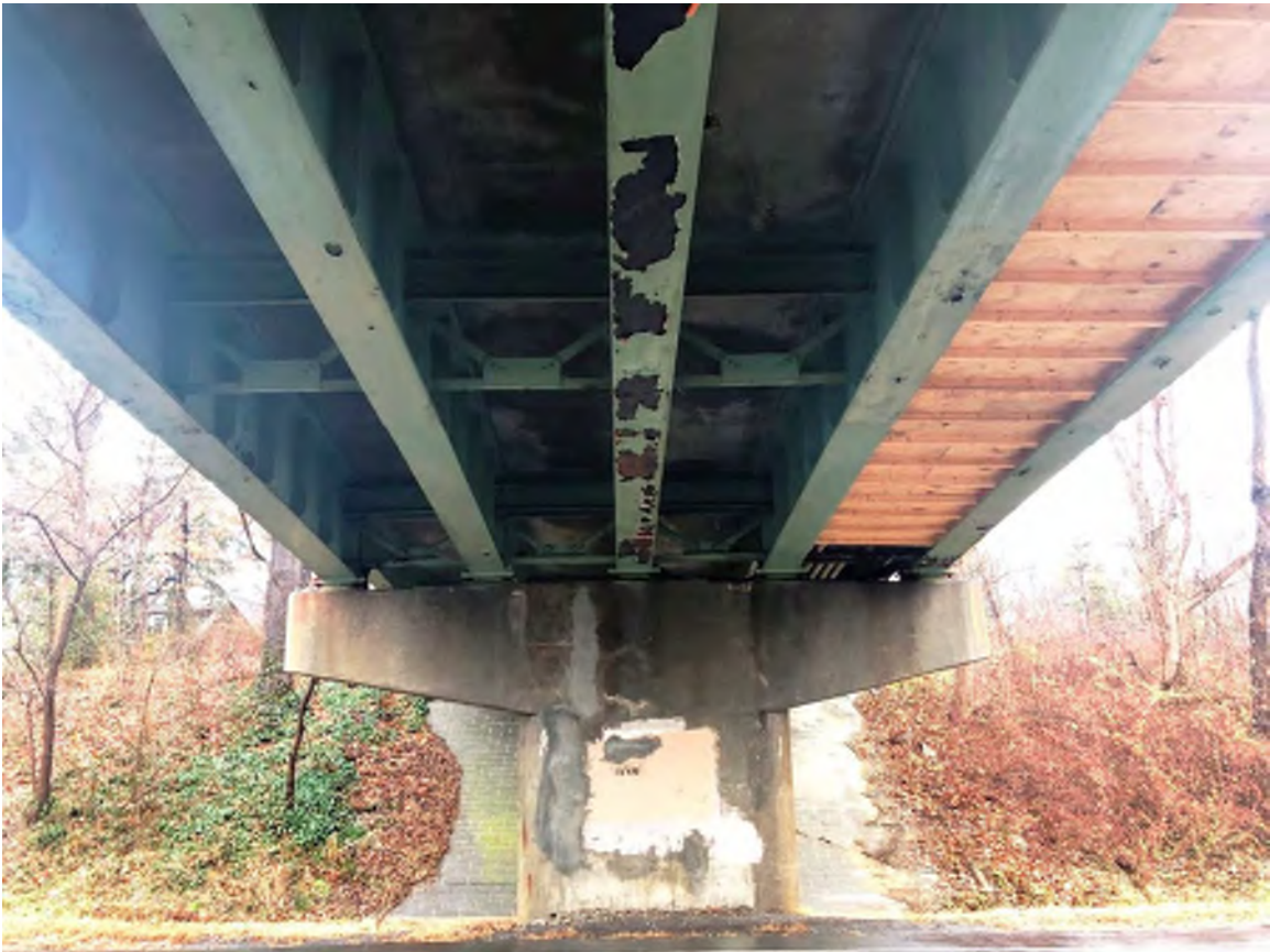
Figure 4 – Existing Bridge Condition Looking North
