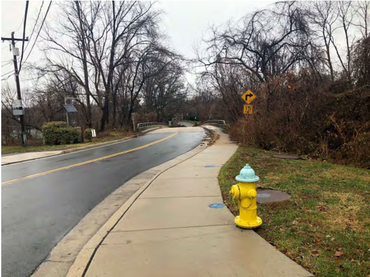
Figure 10 – Underground Utilities on South-East Corner of the Bridge
