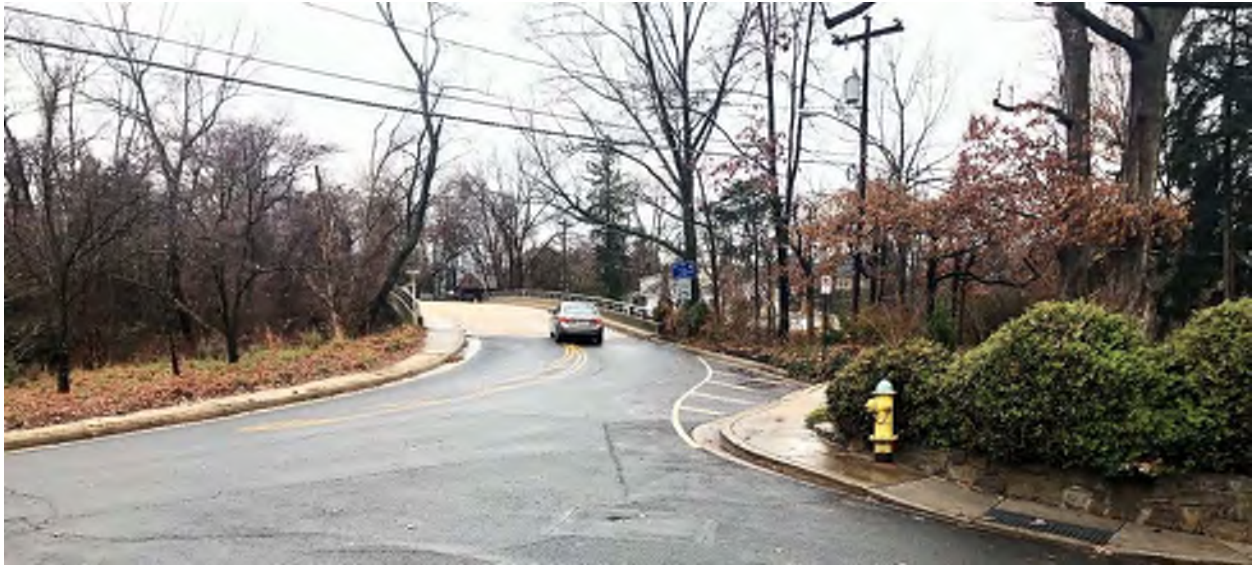
Figure 12 – Underground Utilities on South-West Corner of the Bridge
