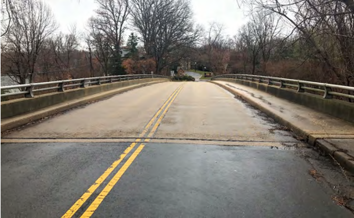
Figure 3 – Existing Structure Looking North
